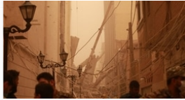
Iran tower-block collapse: 6 dead, dozens injured
